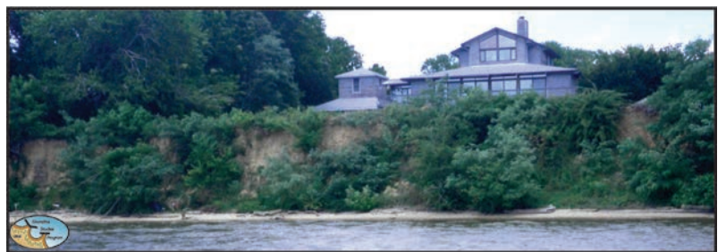
Figure 2-20. Reach 4 erosional bank with no shore protection structures.
