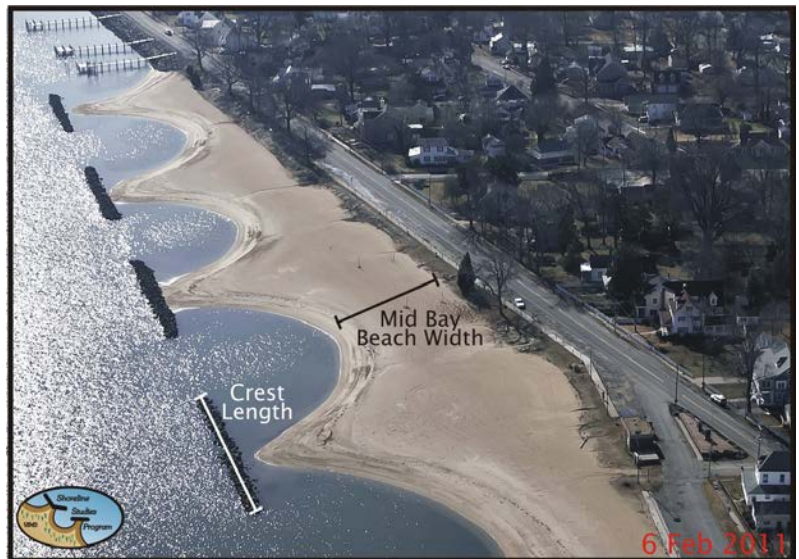
Figure 3-7. The breakwaters at Colonial Beach provide a wide recreational beach as well as storm erosion protection for the residential upland. These structures were installed in 1982.
