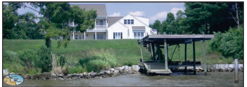
Figure 2-19. Reach 4 low graded bank with shore protection structures.
