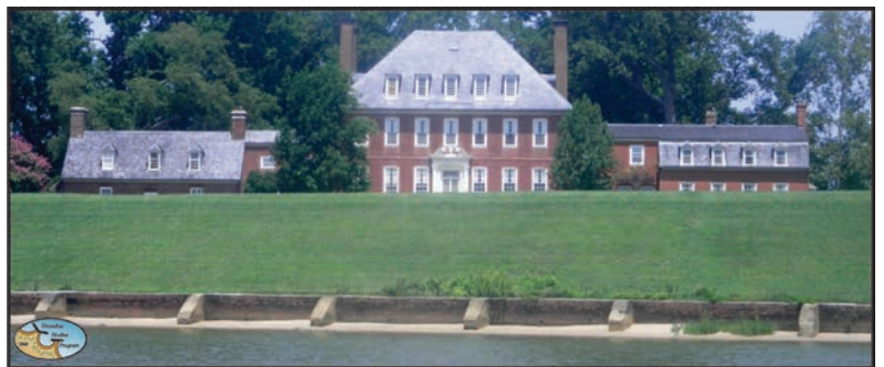
Figure 2-10. Reach 2 bulkhead and short groins at Westover Plantation.
