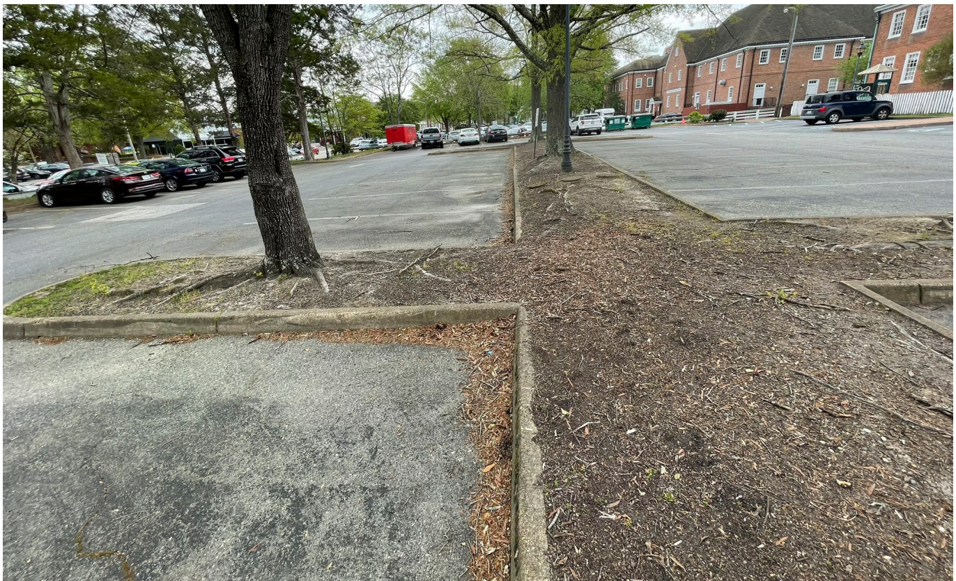
Before photograph of the Williamsburg Baptist Church Parking lot island.
