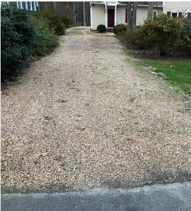
A driveway in James City County including both compacted gravel and concrete slabs adjacent to the garage. The landowners were experiencing issues with excess runoff coming from the driveway, so they chose to replace it with interlocking grid pervious pavers.
